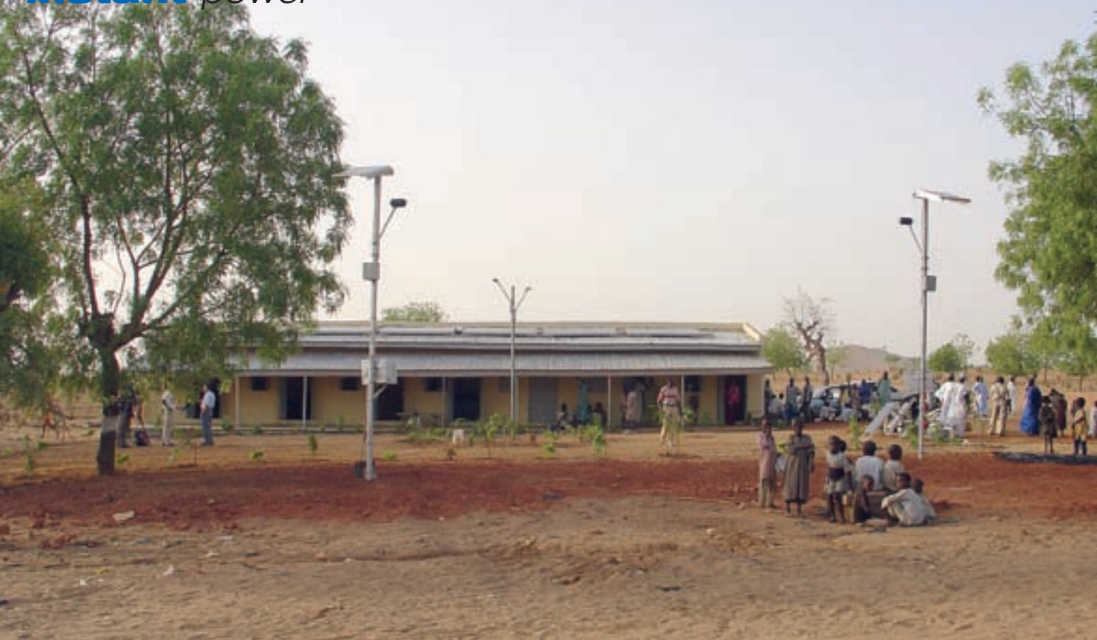
A source of reliable (and clean) electricity supports several small businesses in this microenterprise center.
