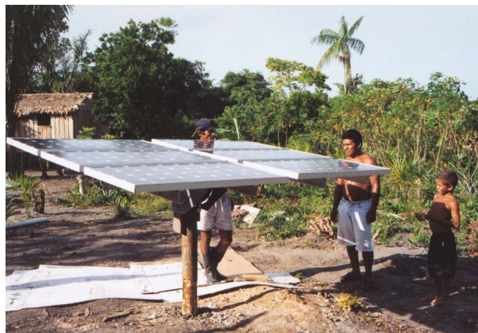
Setting up the solar photovoltaic panel array.
