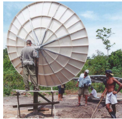
Assembling the satellite dish.
